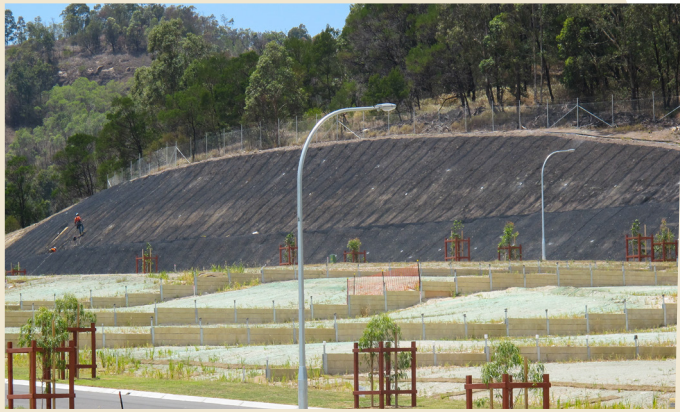
The slope after installation of MacMat R.
