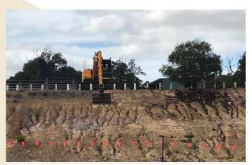
Severe rill erosion from surface run off on the slopes around the hockey field.
